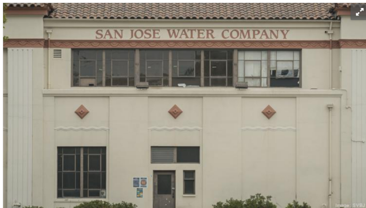
Search giant Google LLC has begun renovating the interior of the historic San Jose Water Company building at 374 W. Santa Clara St. in downtown San Jose to create a new community center. The project is part of Google's Downtown West mixed-use transit village that it's proposed for about 80 acres along the western edge of downtown.
