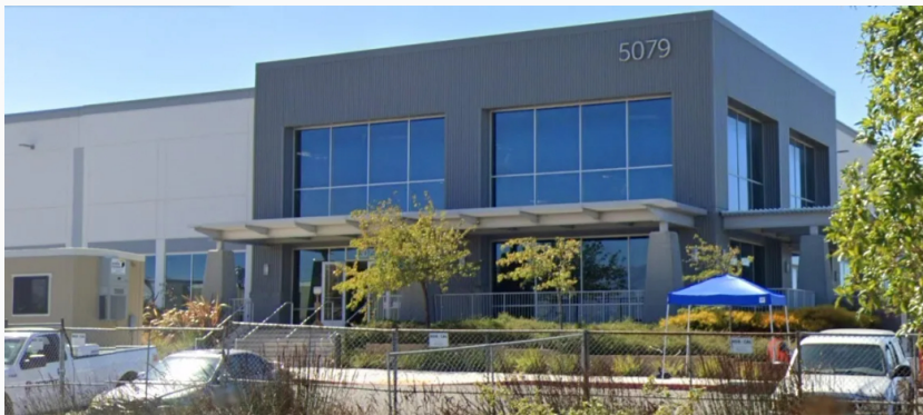
5079 Disk Drive, an advanced research and development building in north San Jose's Alviso district.
